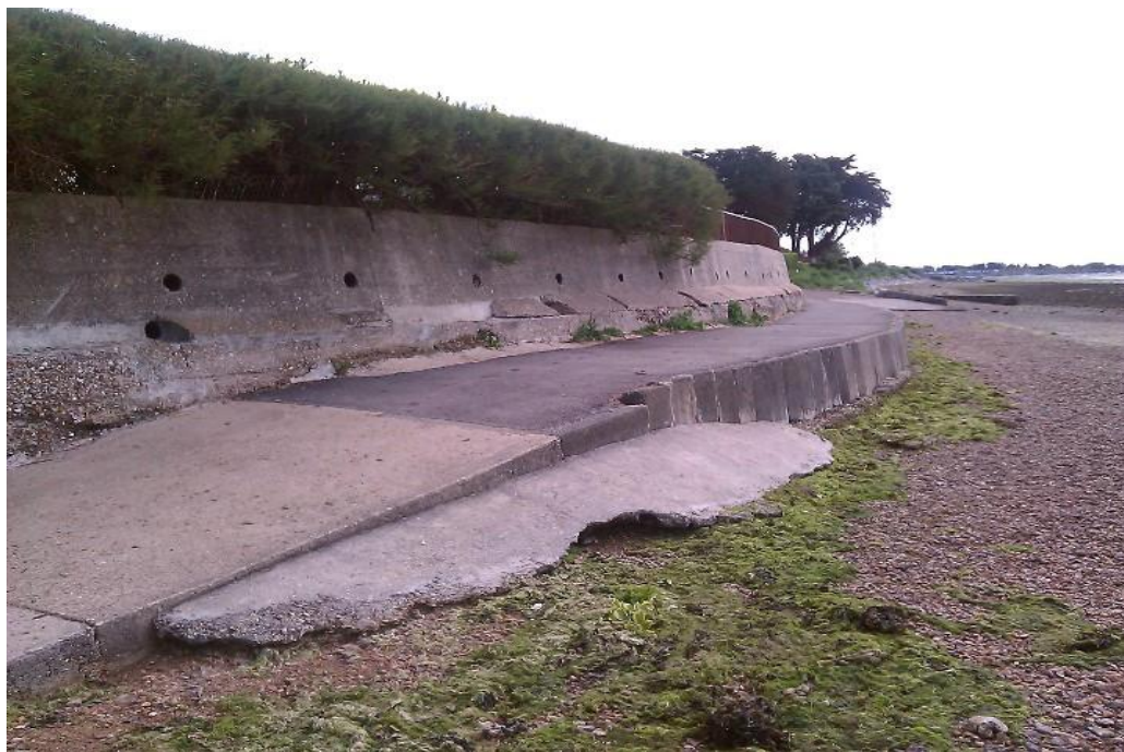
Plate 1: Raised footpath looking South East
