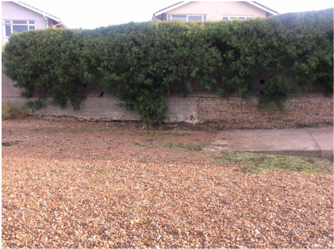
Plate 2: Seawall at foot of access ramp
