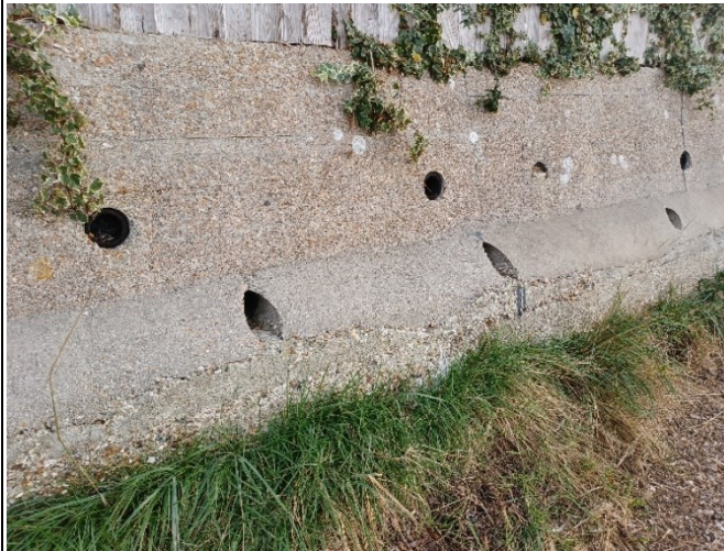
Plate 4: drainage holes in seawall
